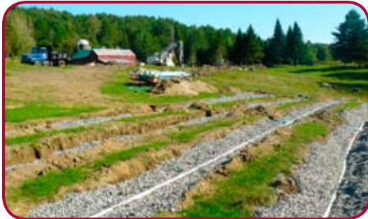
Laying the septic for all future HB buildings!
