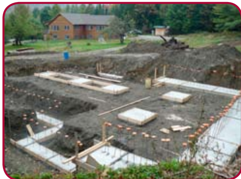
Fourth house foundation pouring has begun!
