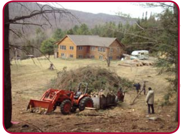
House site clearing
