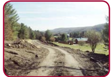
The new road takes shape
